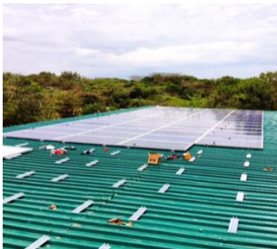
Figure 2: Installation of PV in Kenya (GSOL).
